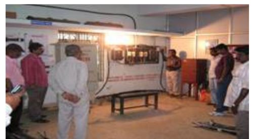
Testing of finished Low Voltage Joint
